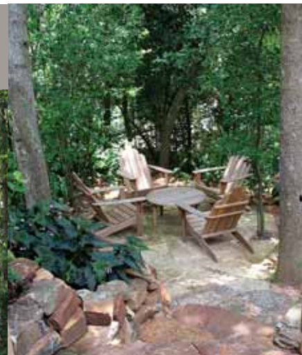
Nestled into the natural area, the lower-level patio was constructed with flagstone and is accessed by steps formed by the placement of large, flat, moss rock boulders.
